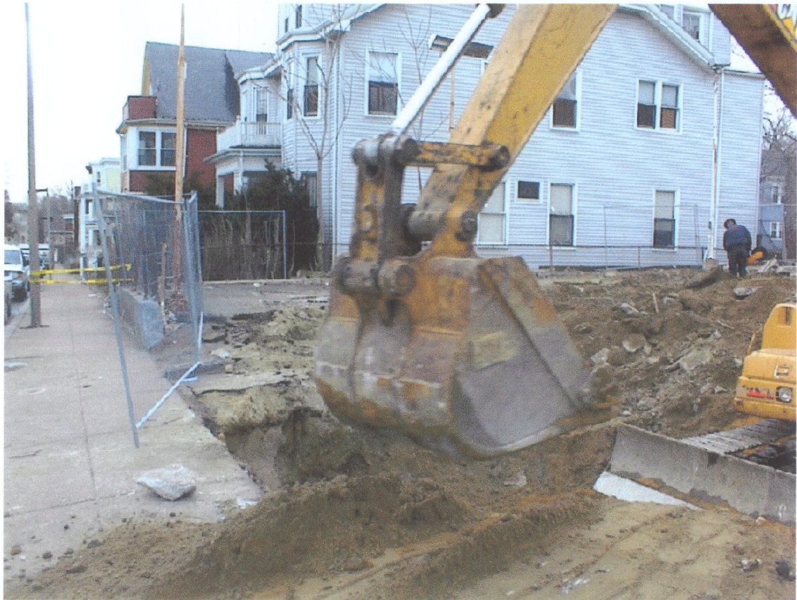
Photo 6: Backfilling process begins: photo taken while facing south on 3/9/06.
