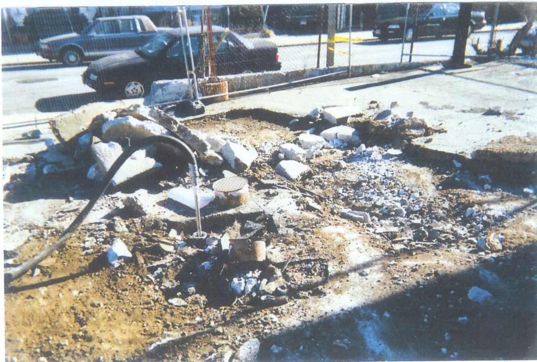
Photo 2: Following the removal of overlying concrete,USTs were pumped out: photo taken 3/7/06.
