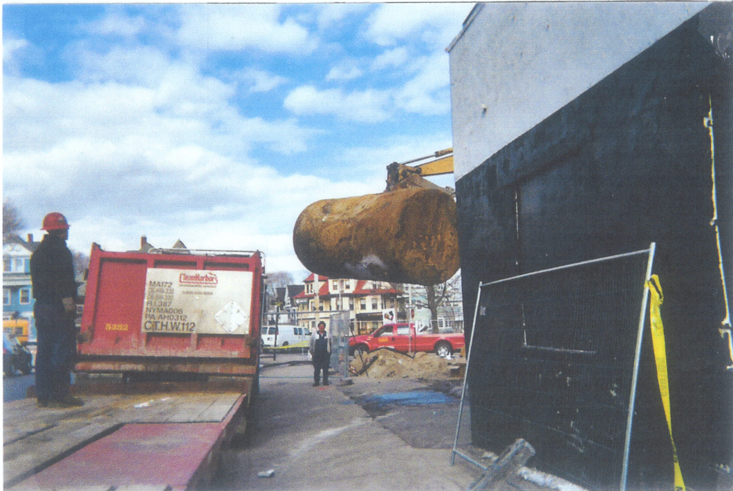
Photo 4: UST is lifted onto flatbed trailer for transport to disposal facility: photo taken facing north on 3/8/06.
