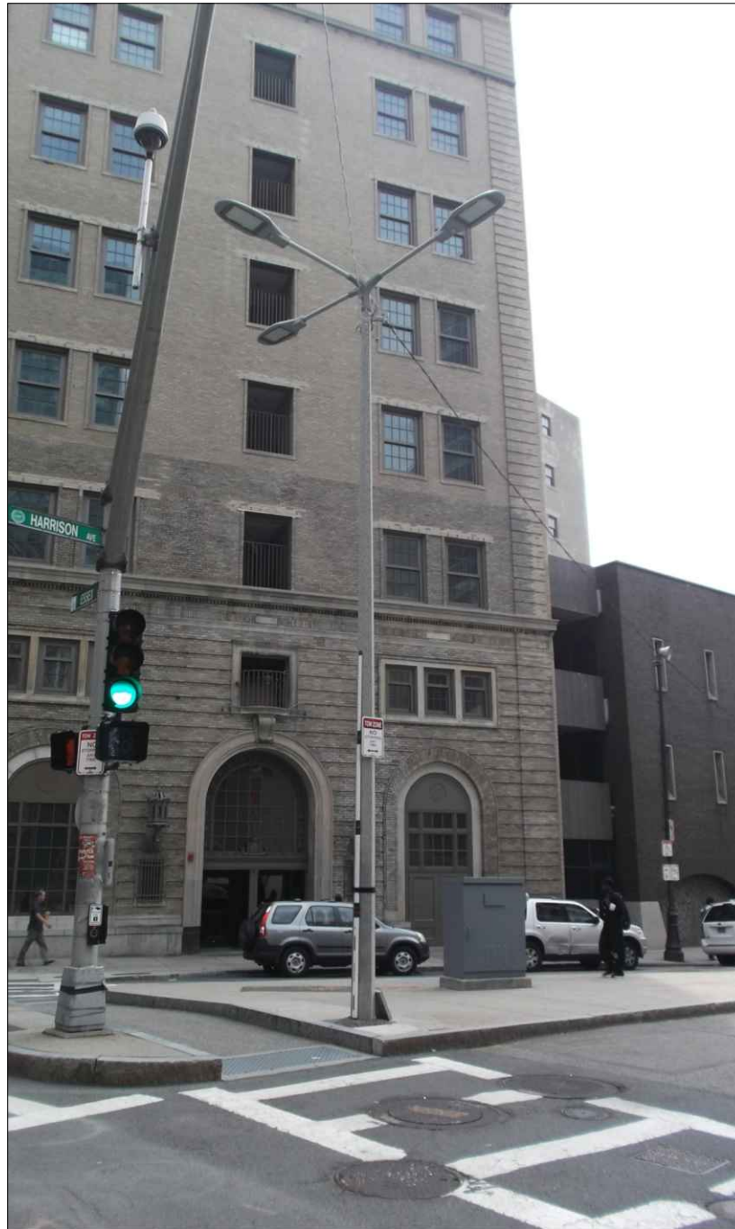
EXISTING PHOTOGRAPHIC VIEW
