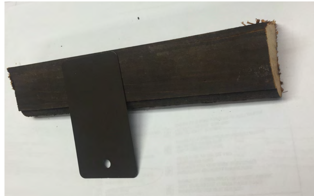
removed brick mold for color match
