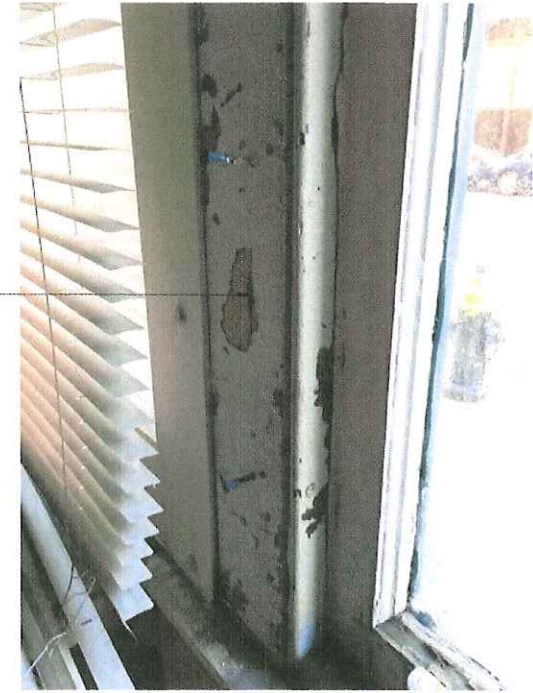
SEVERELY DAMAGED MUNTINS
