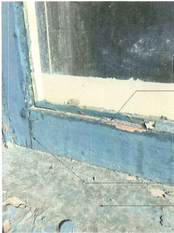
DAMAGED + ROTTING WOOD SHELF
