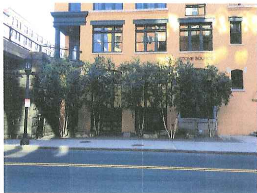
327 A ST - GRAVEL/PLANTING AREA
