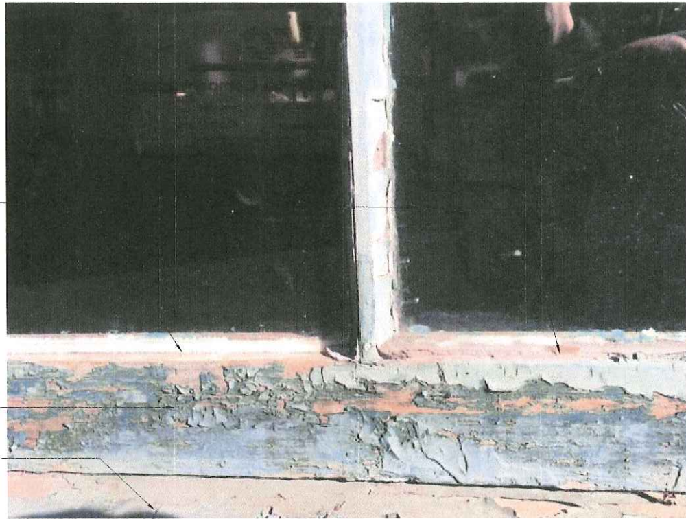
DAMAGED + ROTTING WOOD SHELF
