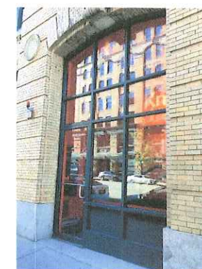
281 SUMMER ST (SAME BUILDING)
