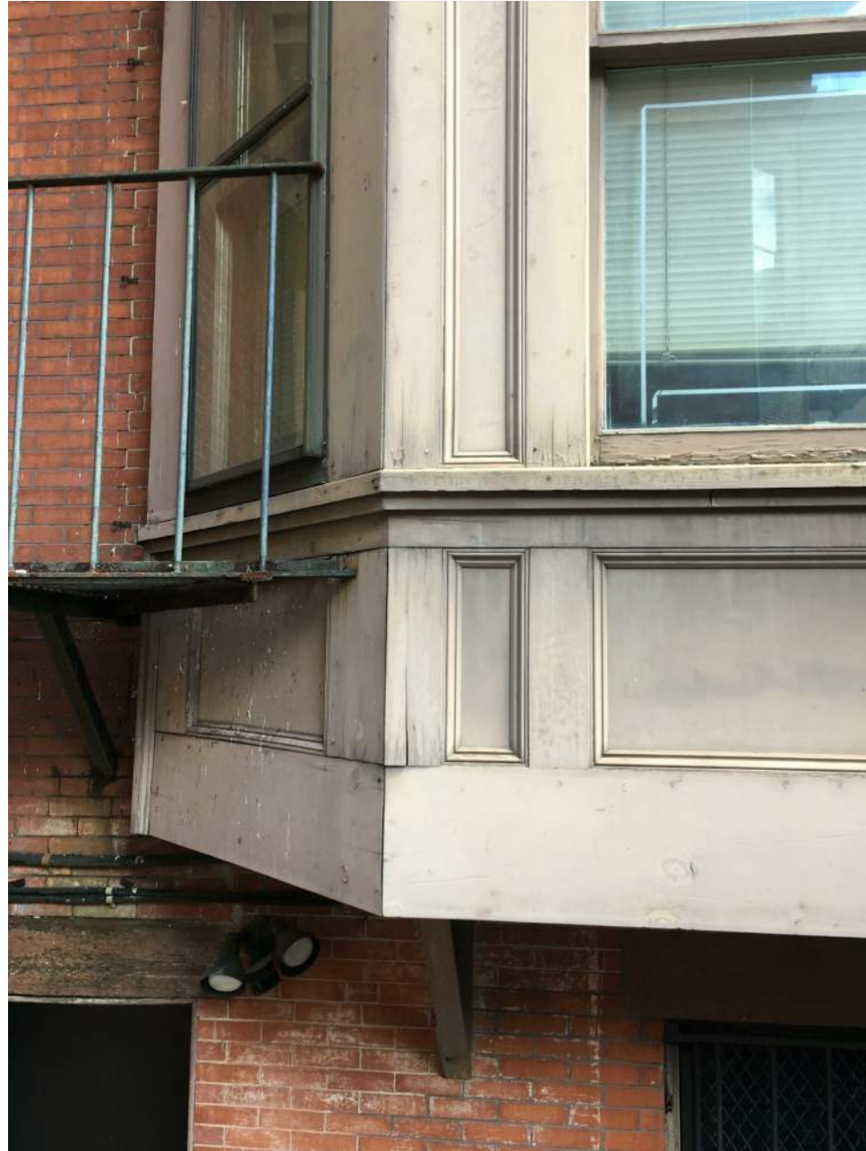
EXISTING NON-HISTORIC ORIEL SUPPORTED ON METAL BRACKETS
