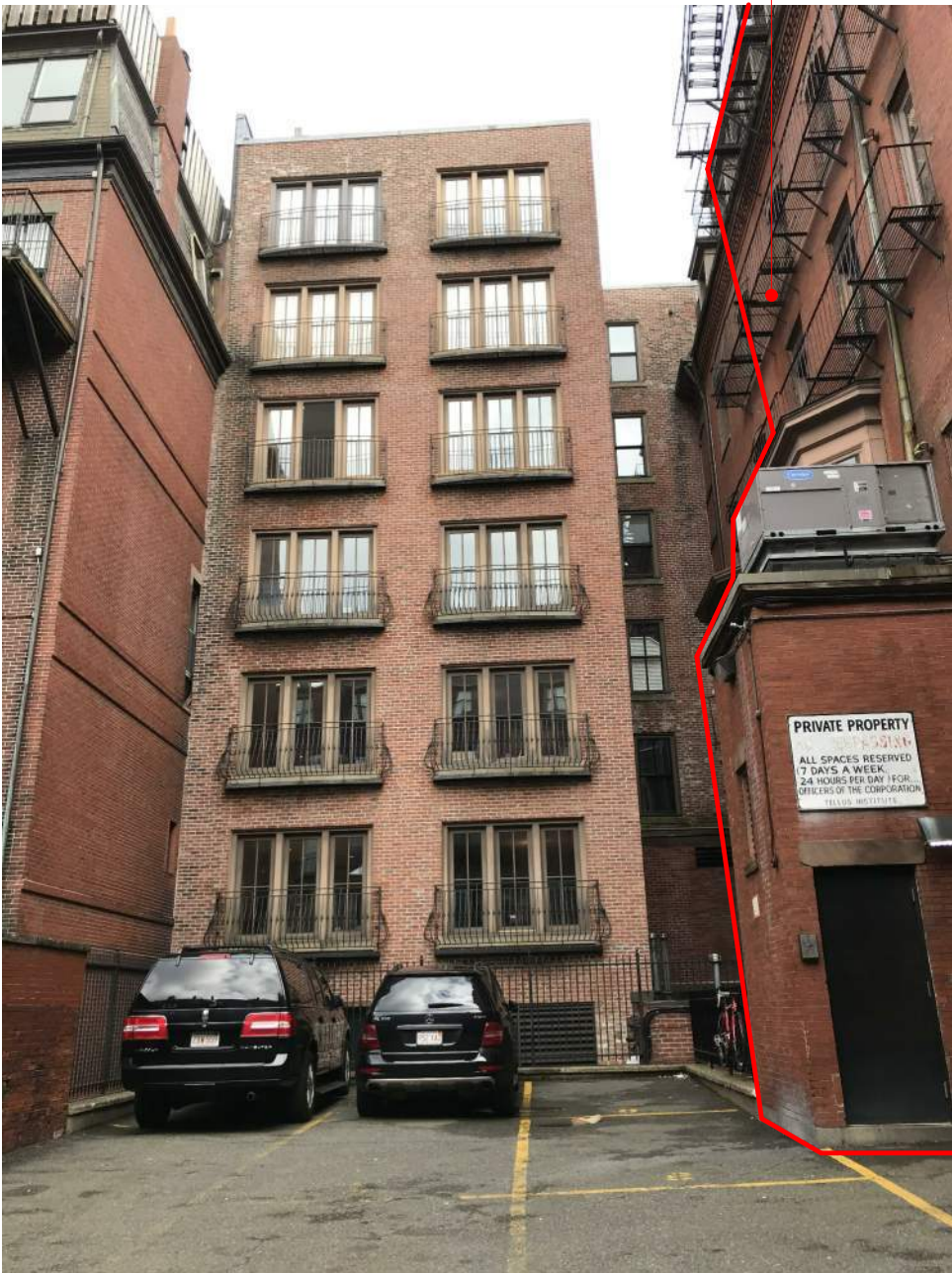
ALLEY CONDITION AT REAR OF 10-11 ARLINGTON STREET
