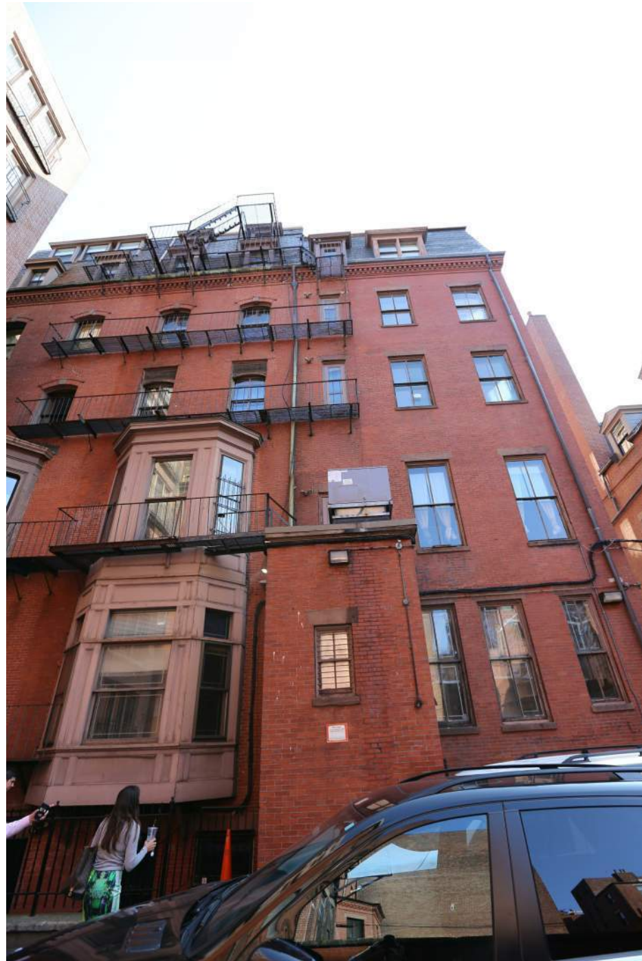
REAR FACADE - 10-11 ARLINGTON STREET
