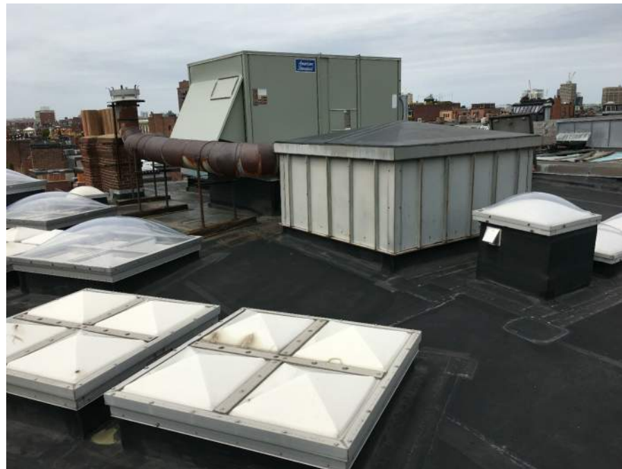
VIEW FROM SE CORNER OF 10-11 ARLINGTON STREET LOOKING NW
