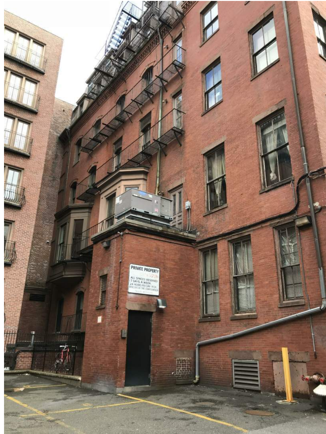
REAR FACADE - 10-11 ARLINGTON STREET
