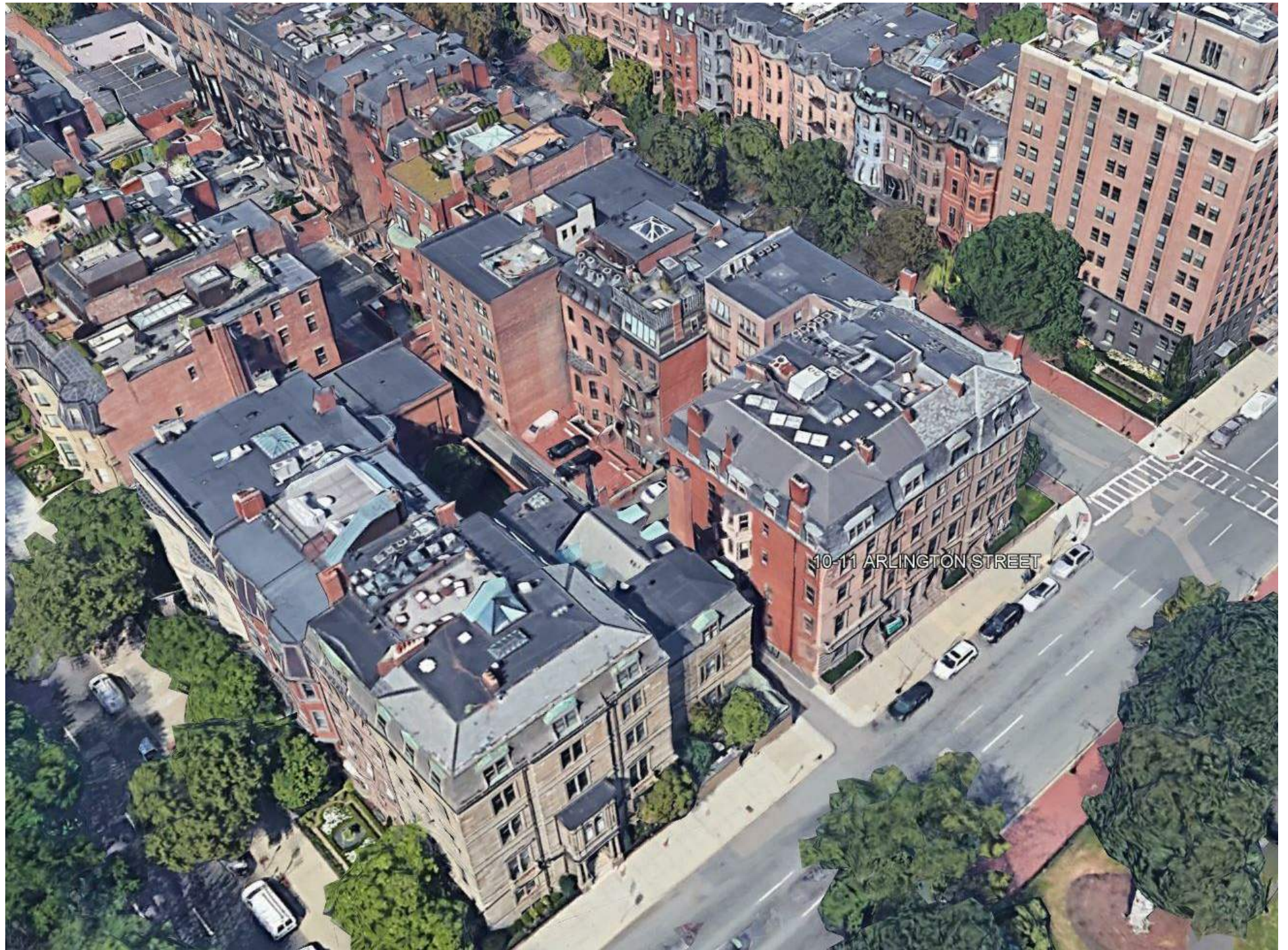
OVERHEAD VIEW OF 10-11 ARLINGTON STREET LOOKING NORTHWEST
