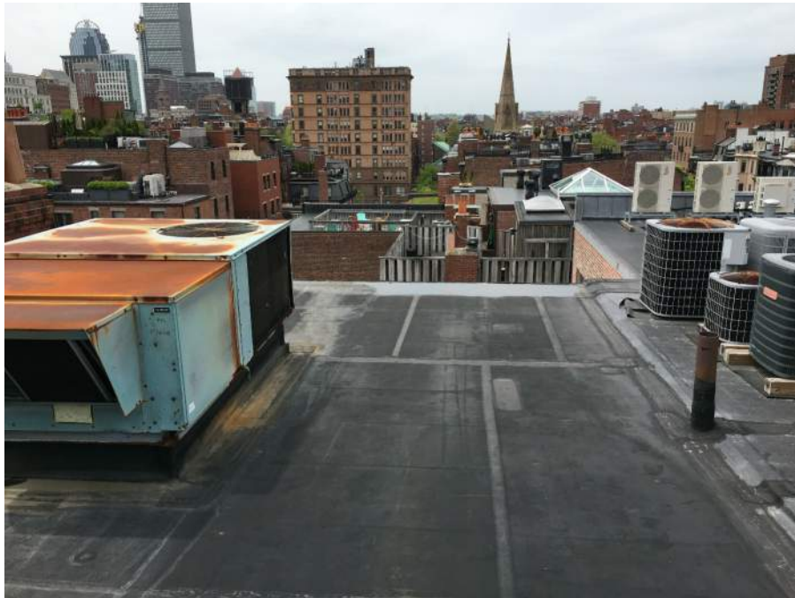
VIEW FROM MIDROOF OF 10-11 ARLINGTON STREET LOOKING WEST
