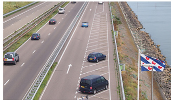
Example: Afsluitdijk Roadway, Netherlands. Designed by Zuiderzee Works.
