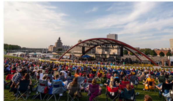
Example: Cedar Rapids Riverfront Multi-Purpose Levee, Cedar Rapids, Iowa. Designed by Sasaki.
