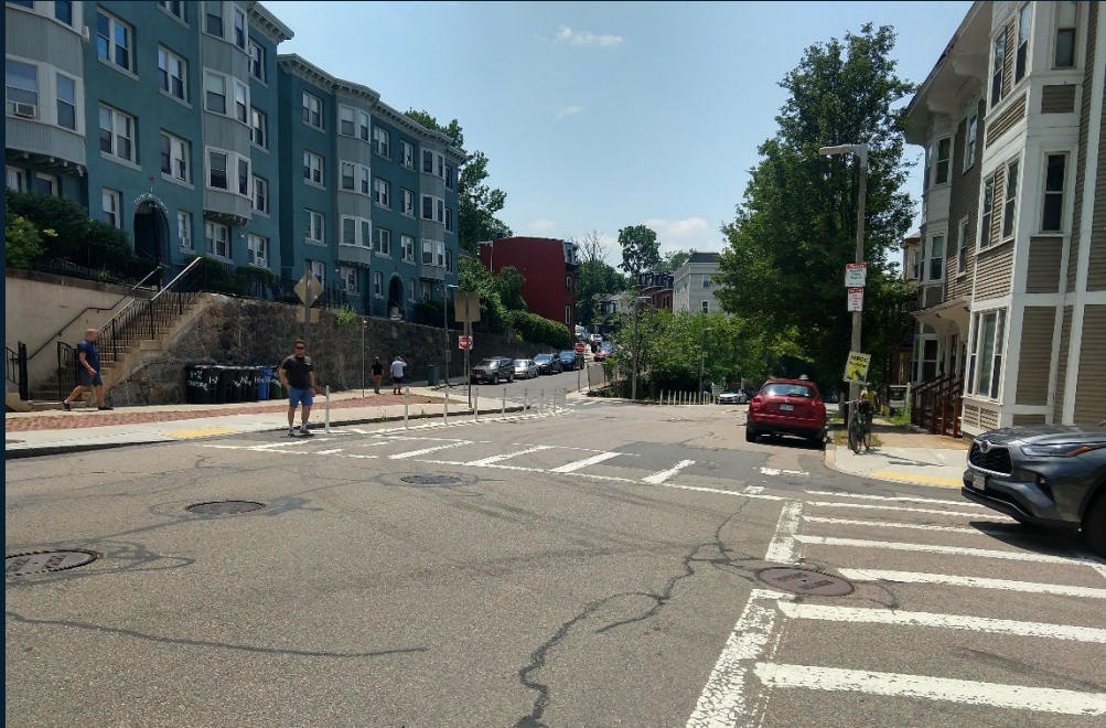
New crosswalk and accessible ramps Parking restrictions with paint and flex posts
