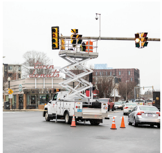
2021 powerline repairs Allston
