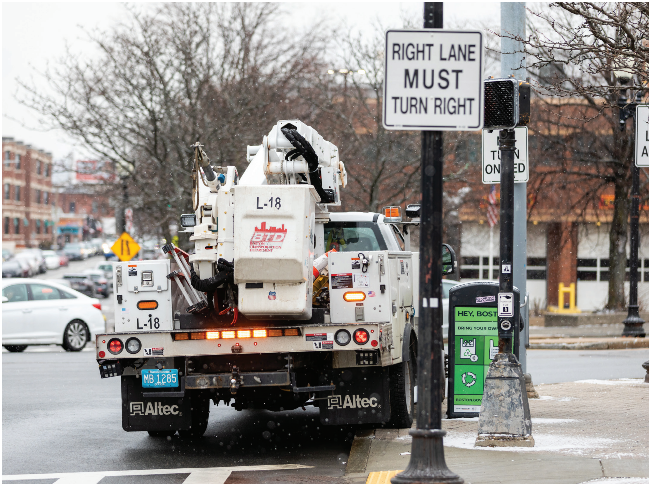
2021 Allston Power Line Repair
