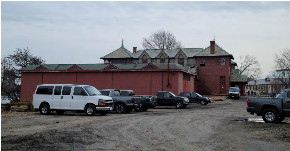
7. Newell Boathouse addition from driveway at Soldiers Field Road. Addition in front, with historic boathouse in background. (3-7-22)
