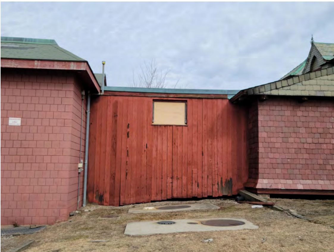
2. Newell Boathouse addition connector. Addition at left, historic boathouse at right. (3-7-22)
