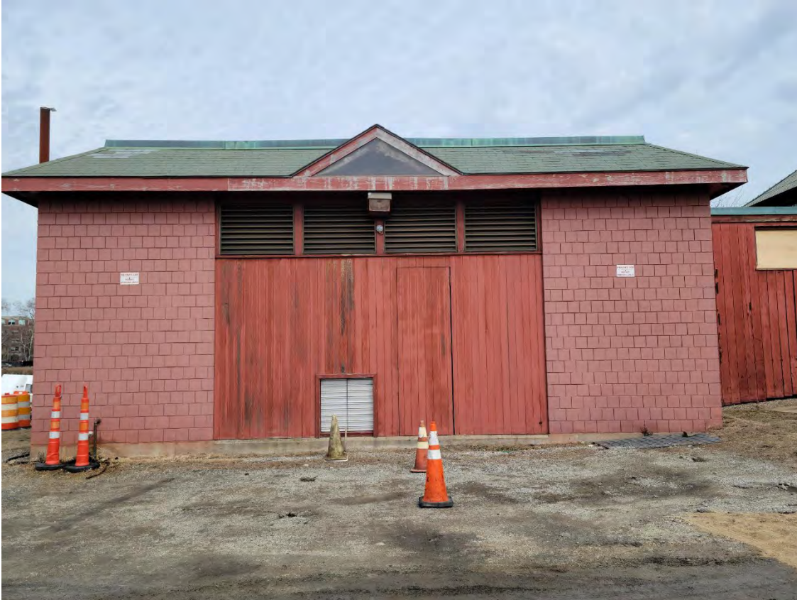
1. Newell Boathouse addition southwest façade. (3-7-22)
