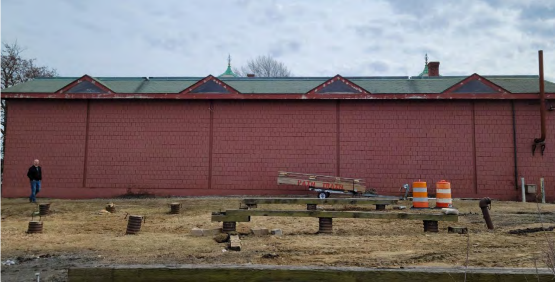
3. Newell Boathouse addition northwest façade. (3-7-22)
