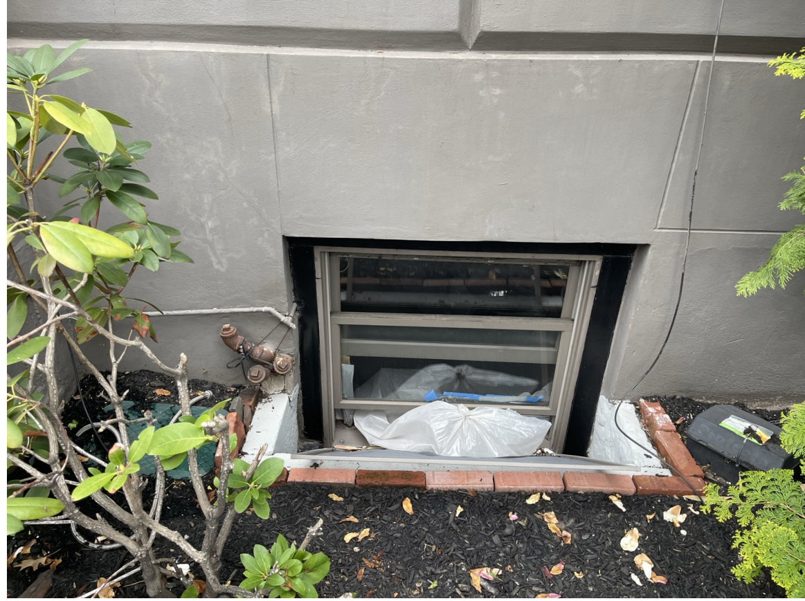
LEFT BASEMENT WINDOW
