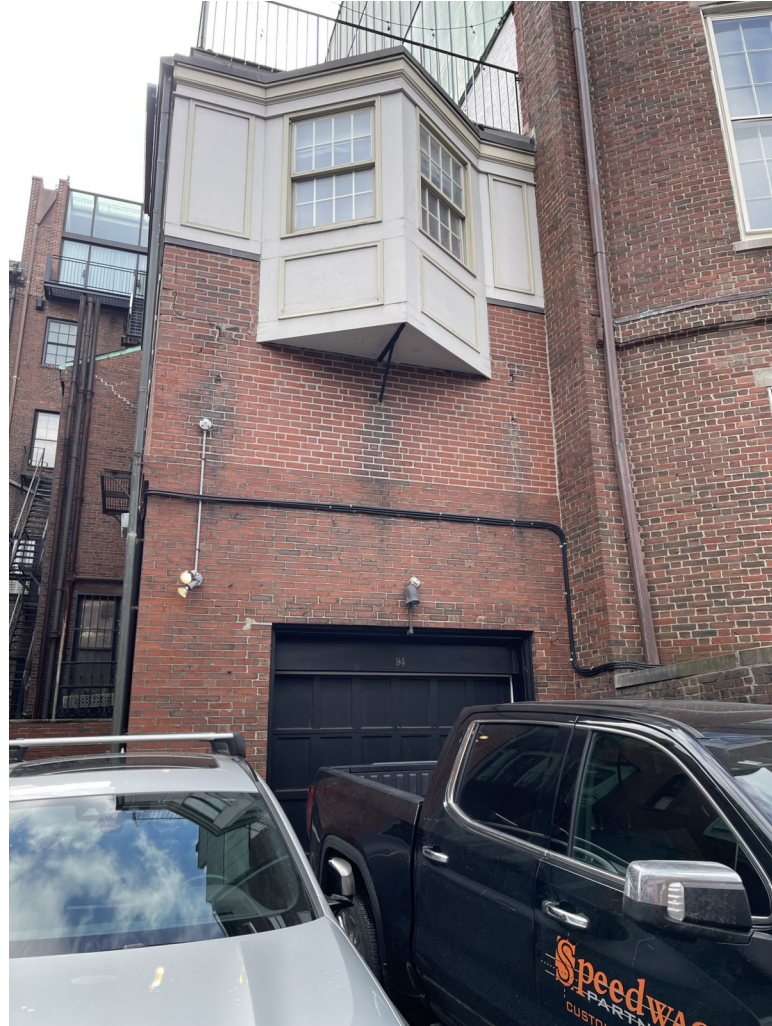
EXISTING GARAGE DOOR LOCATED ON BEAVER PLACE
