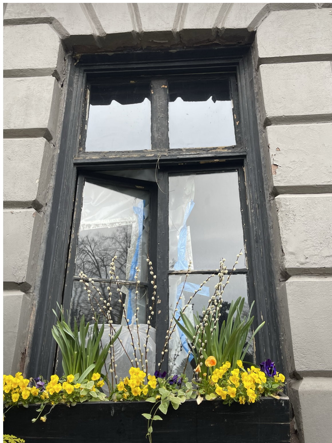
FIRST FLOOR FRENCH CASEMENT
