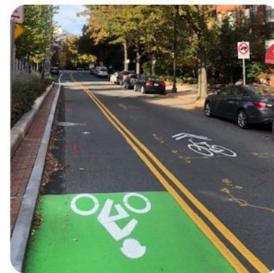
Contraflow bike lane
