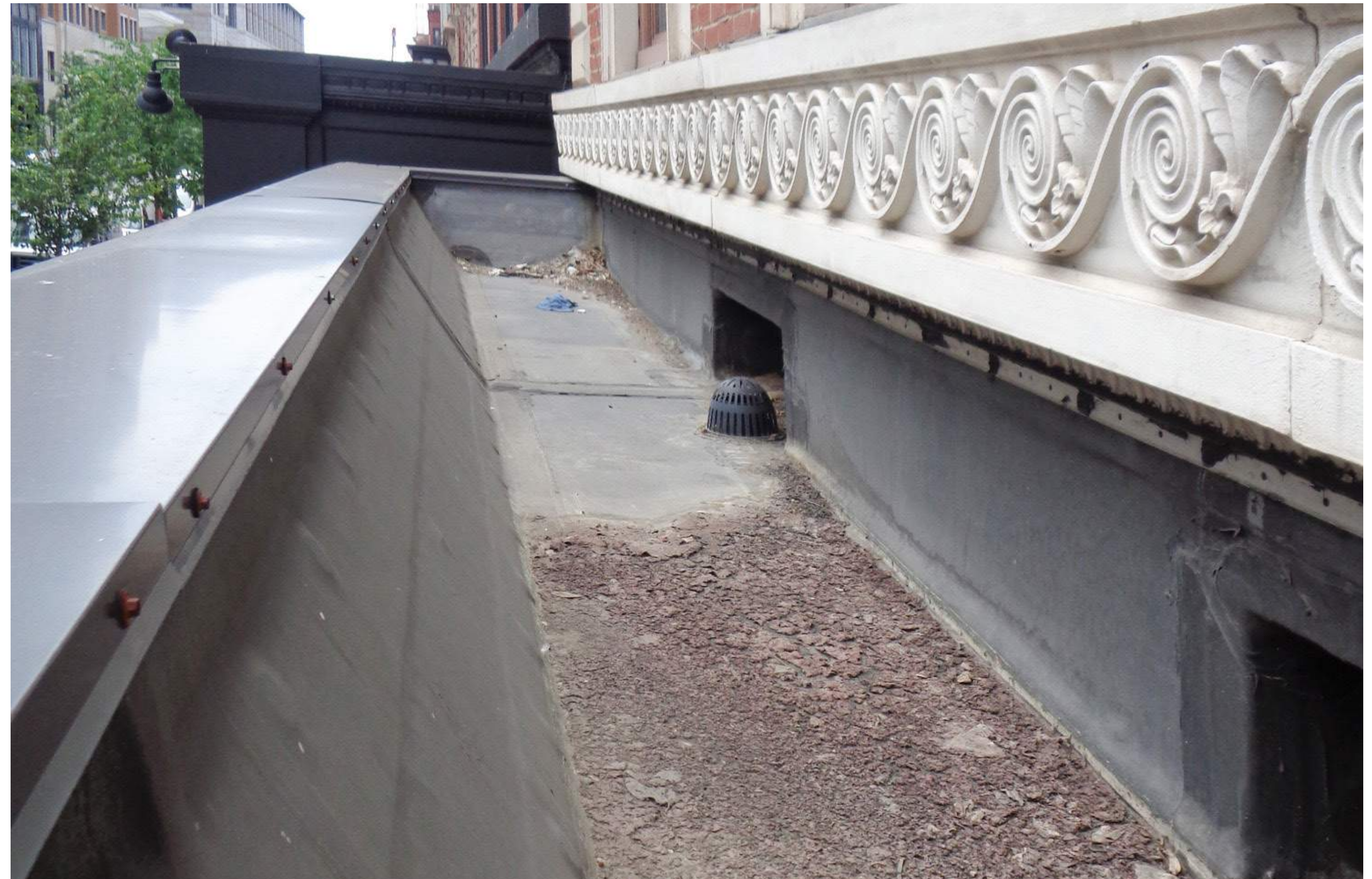
Existing Max Brenner Roof and Roof Drain Conditions
