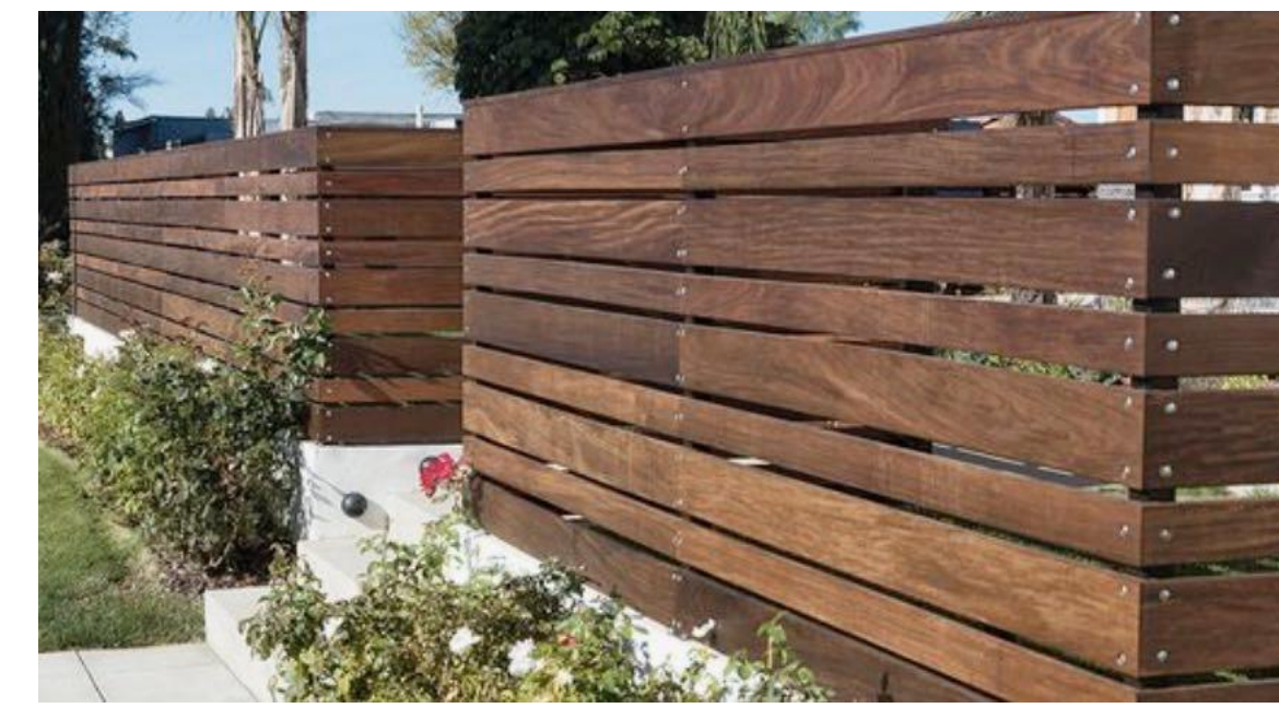
6" HARDWOOD GUARD RAILS, STD., THROUGH-BOLT TO PTD. STL GURD POSTS
