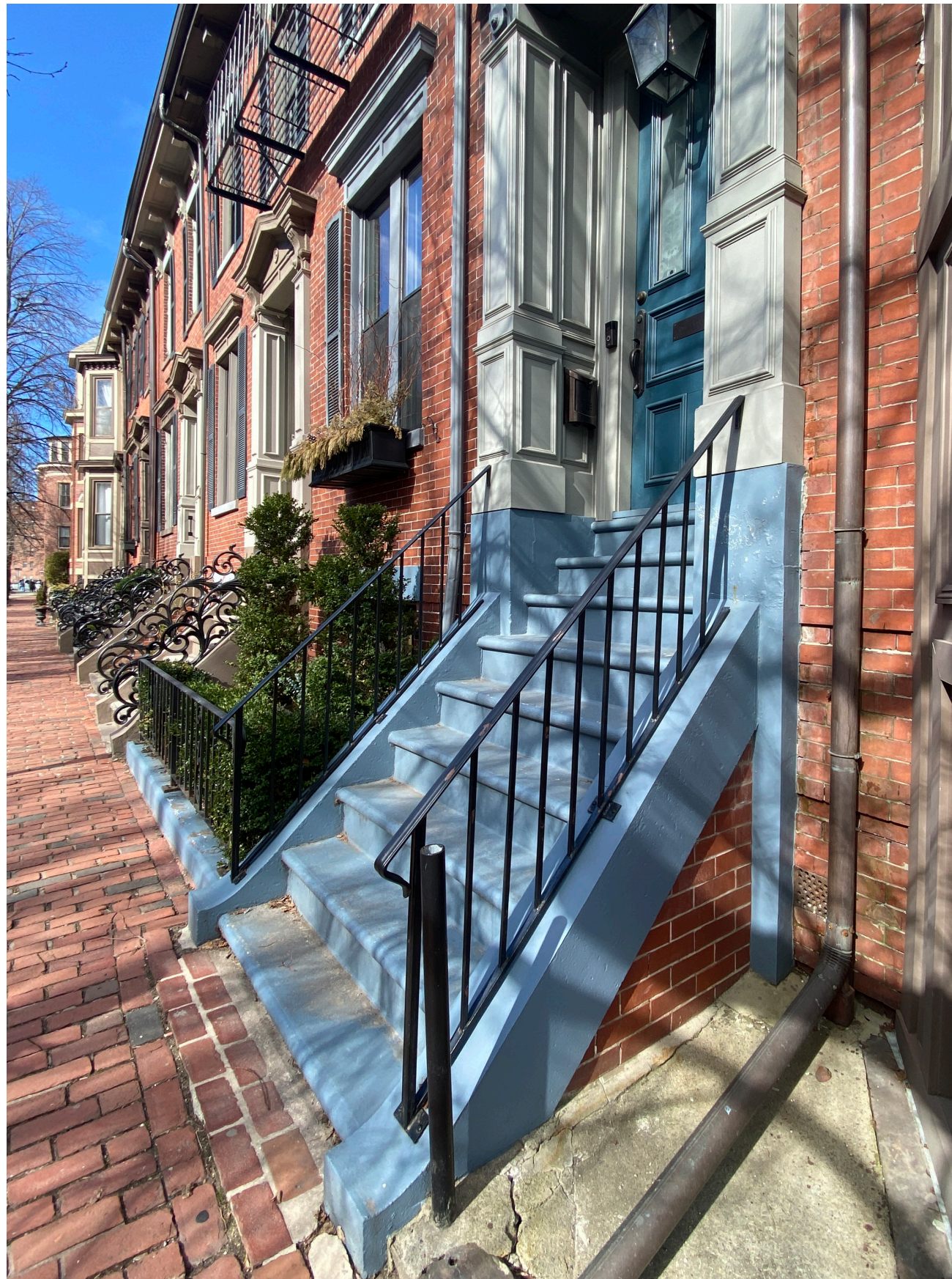
Existing Front Stairs Railing
