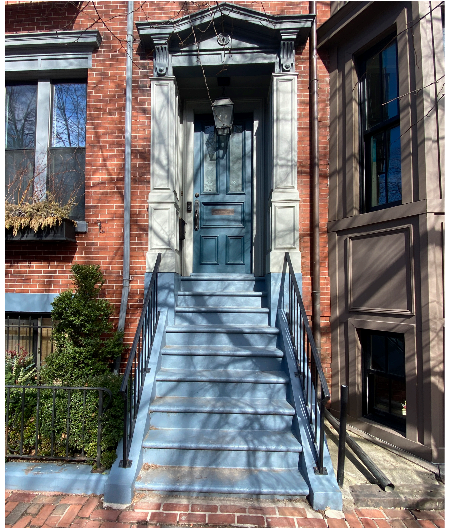
Existing Front Stairs Railing
