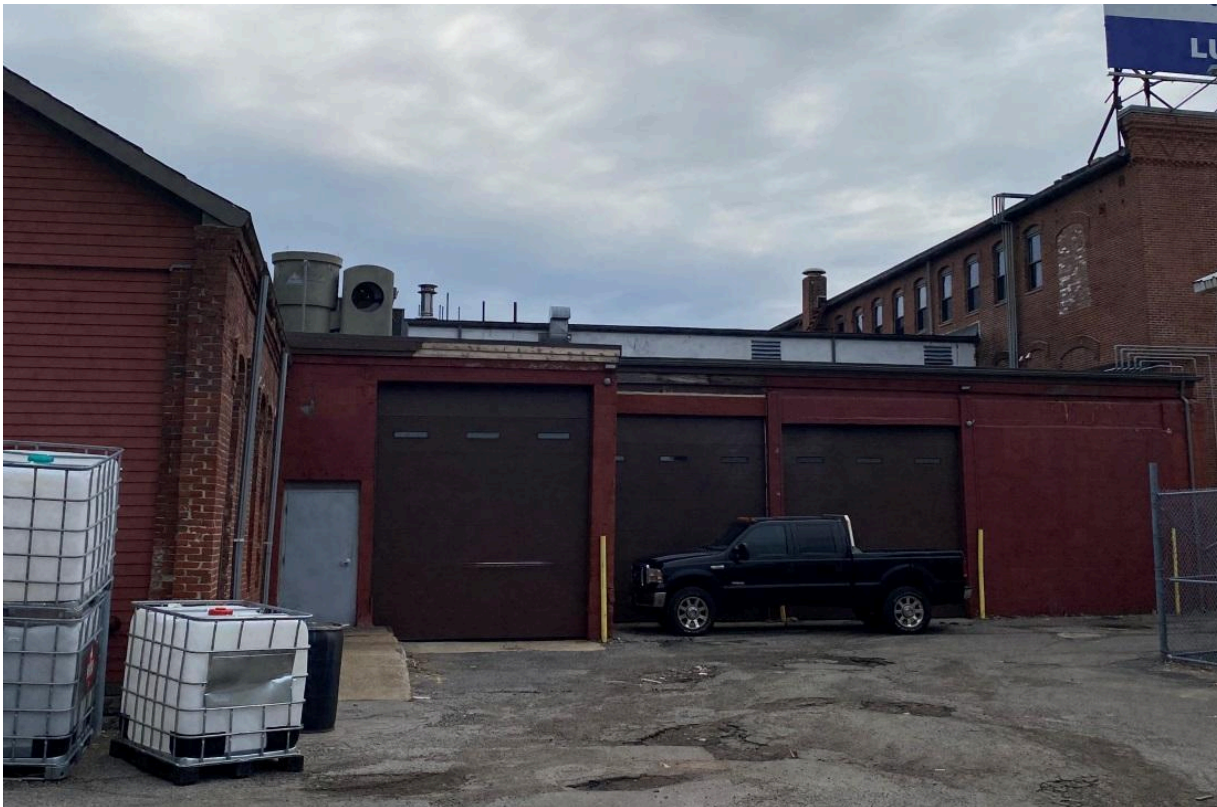
Figure 10. West-facing side showing the pass-through structure connecting 12 and 12R Ericsson St. Photo by John D. Clemson, March 17, 2023.
