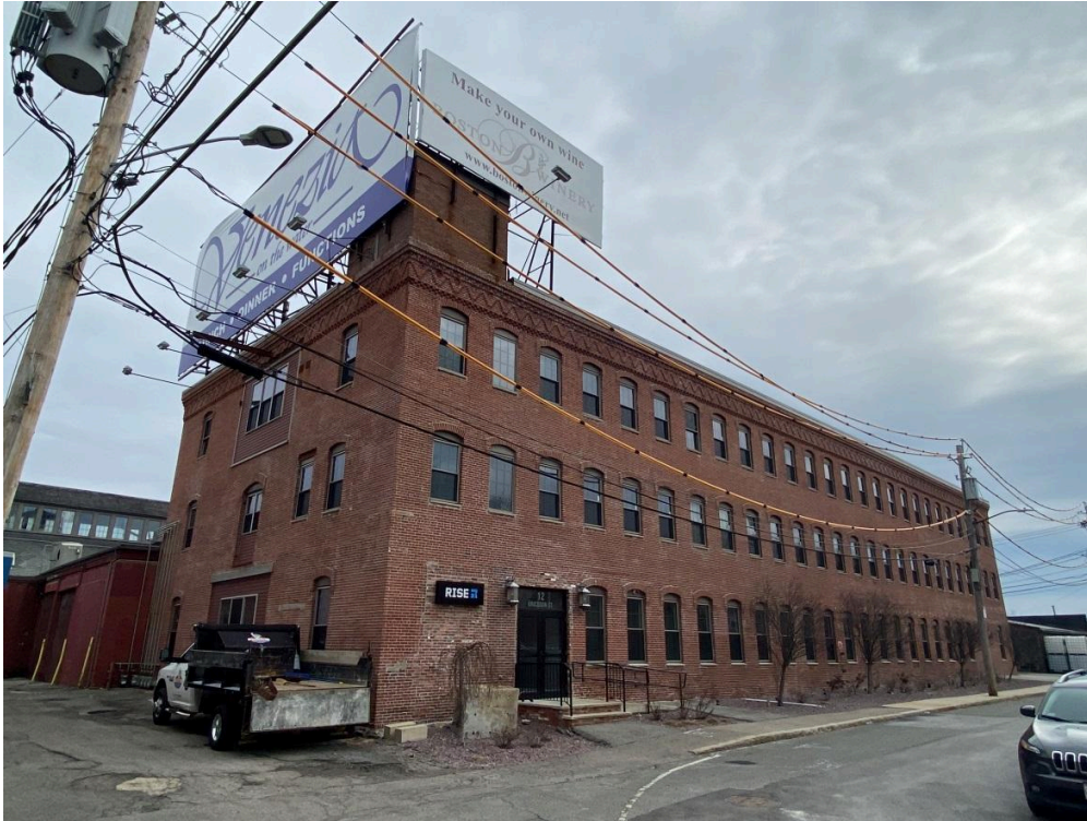
Figure 3. 12 Ericsson St. showing west-facing side elevation. Photo by John D. Clemson, March 17, 2023.
