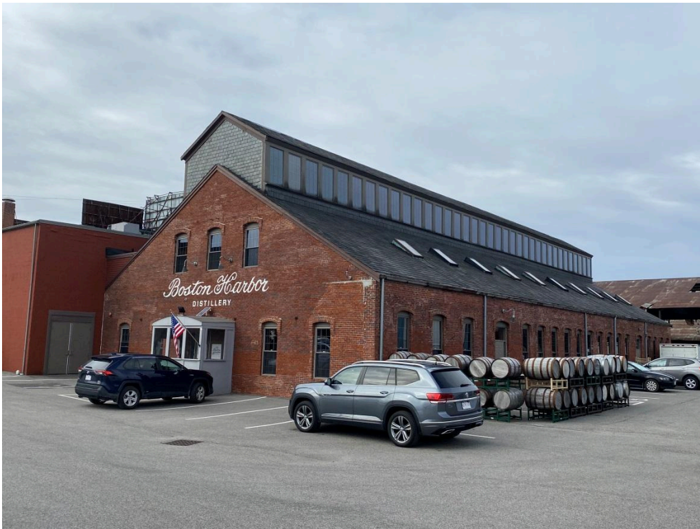
Figure 7. 12R Ericsson St. showing east- and north-facing elevations. Photo by John D. Clemson, March 17, 2023.
