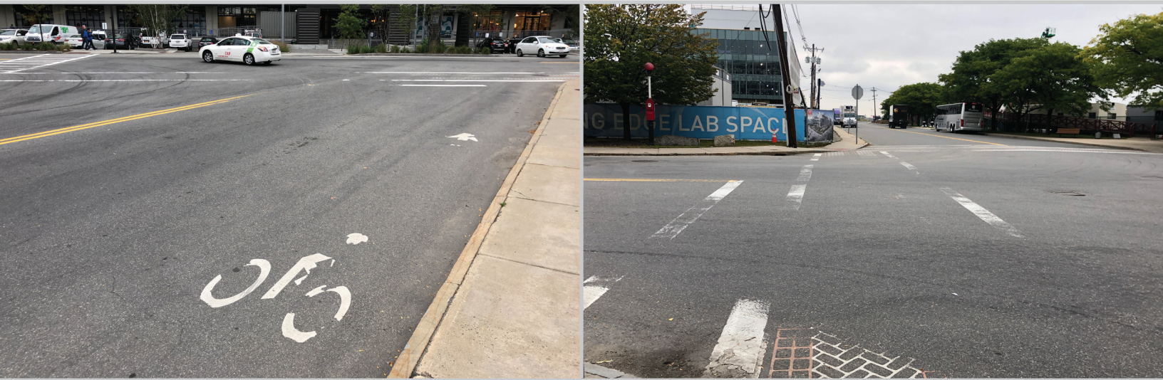
(LEFT) Bike lane markings along Tide Street. (RIGHT) Stop lines and pedestrian crosswalk along Northern Avenue.
